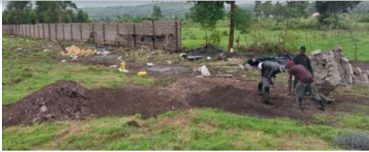
Builders constructing the Security wall at Act High School.
