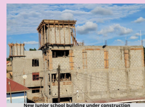
New Junior school building under construction
